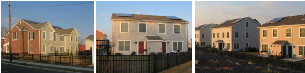
Twenty-two 1.11 kW systems – Philadelphia Housing Authority (left: Brown Street; center and right: Mifflin Street)
