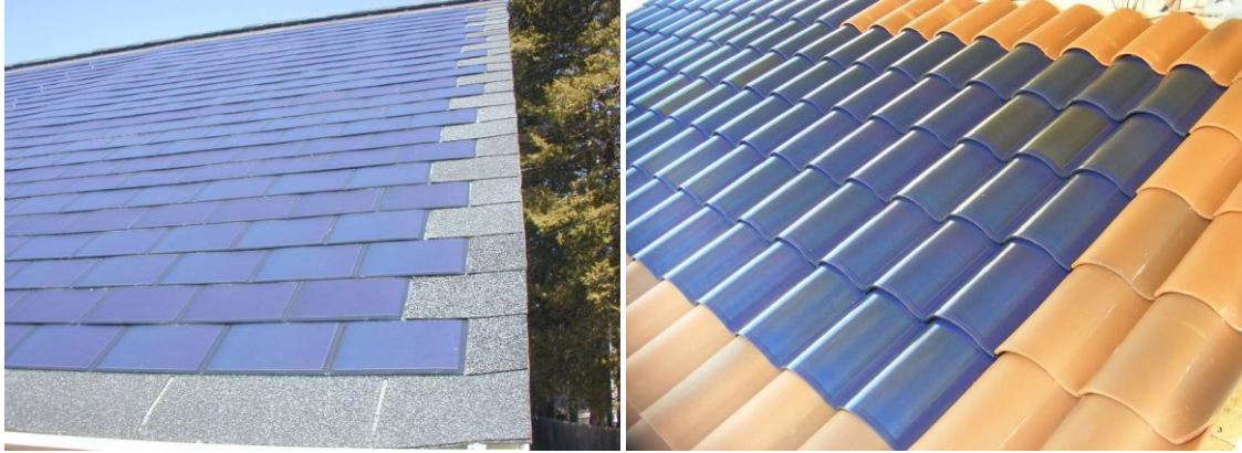
Figure 2-4: PV modules integrated into roofing materials (left: Uni-Solar roof shingles; right: SRS Energy Solé Power Tile roof tiles)
