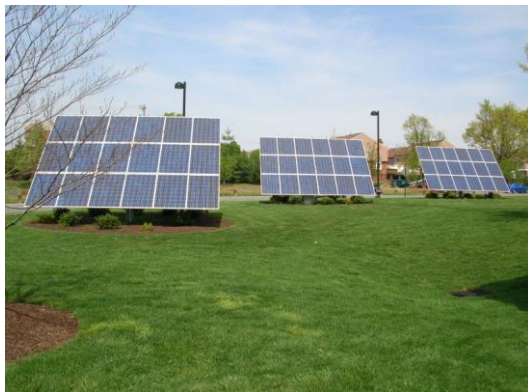
Figure 2-10: Ground Mounted PV System (Three Eagles-Nova Care)
