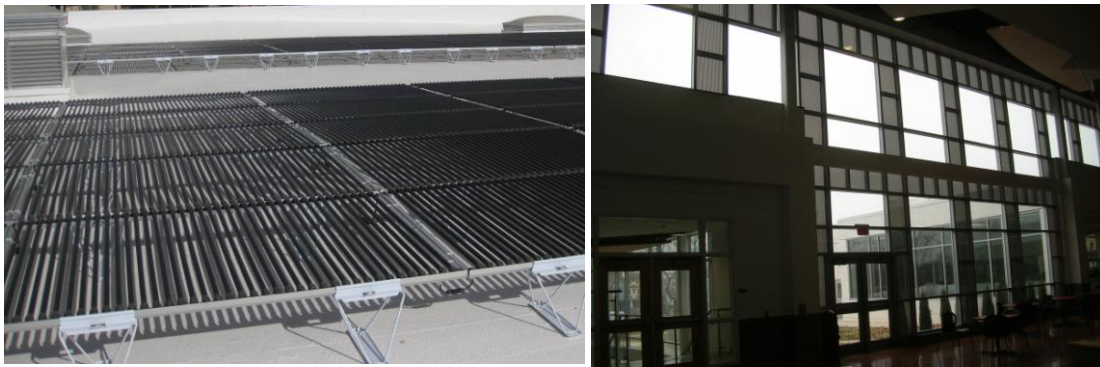
Figure 2-5: Cylindrical PV Cells by Solydra, Inc. Source: City of Tucson, Solar America Cities Program
