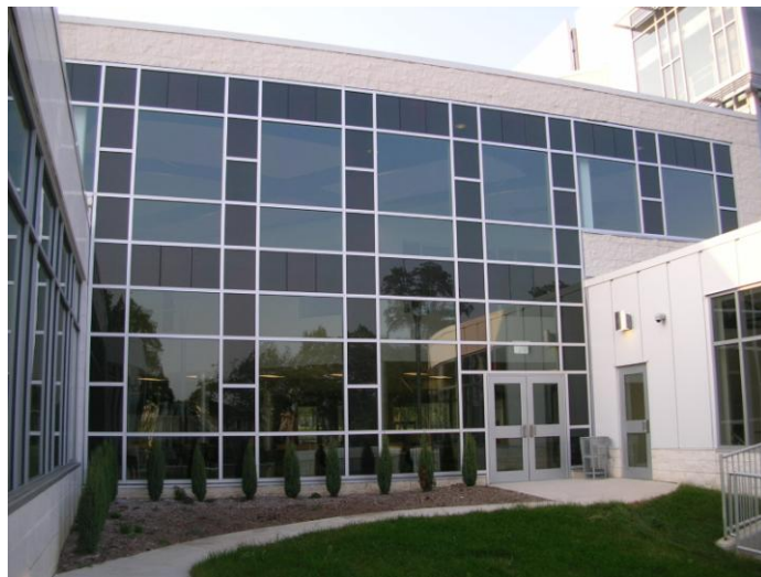
Figure 2-3: BIPV example, PV modules integrated into windows, Microsoft School, Philadelphia Source: Celentano Energy Services
