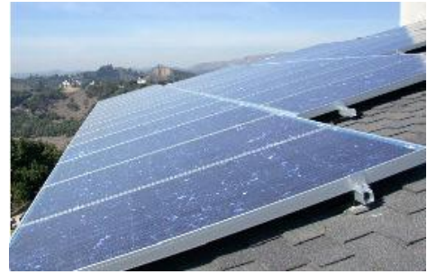
Figure 2-8: Integral mounting system for rooftop (attach directly to roof rafters)
