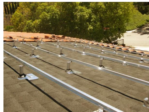
Figure 2-9: Standoff mounting system for rooftop (several inches off the roof surface allowing natural venting)
