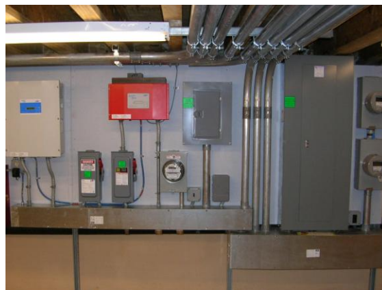
Inverter, electric panel and disconnects (IBEW 98 – South Philadelphia)
