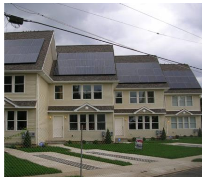
Staggered Row Homes each 3.13 kW PV, Northeast Philadelphia
